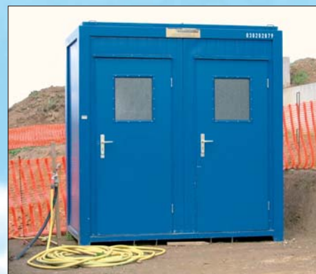
WC cabin on a building site
